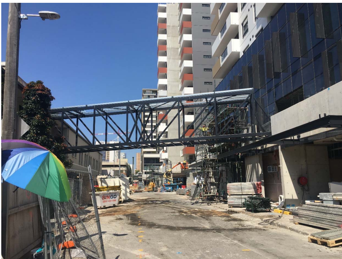
Image 4: The link bridge between the buildings under construction over the laneway.
